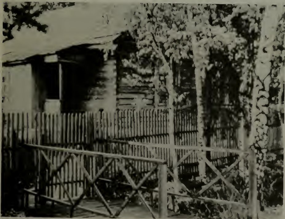
A wooden ward building at Mental Hospital #14.
